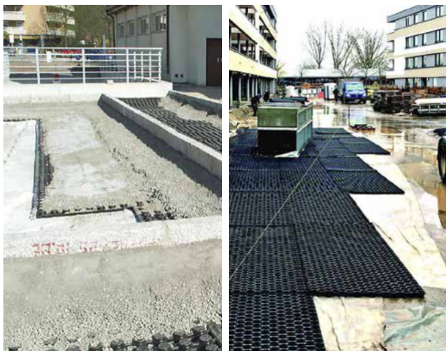
BauderGREEN DSE 40 drenaaži paigaldamine
