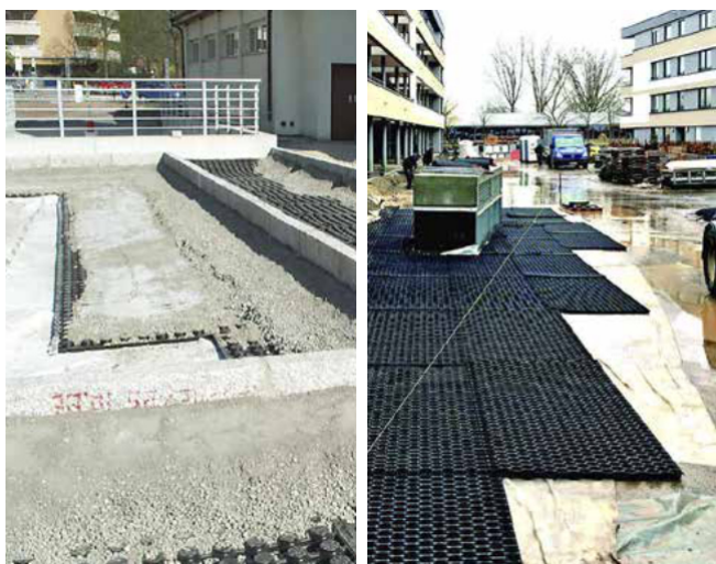
BauderGREEN DSE 40 drenaaži paigaldamine
