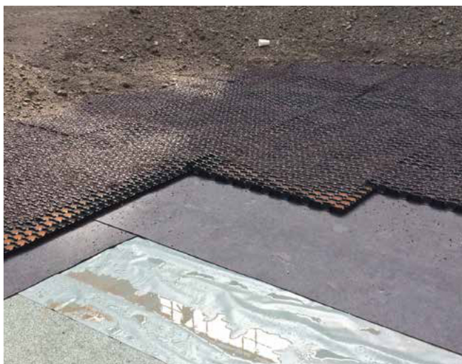
BauderGREEN PE 02 ja BauderGREEN FSM 600 paigaldamine
